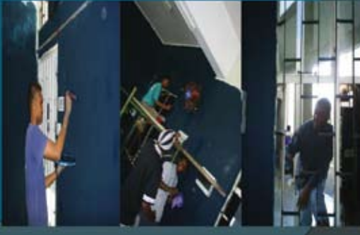
Painting of walls
